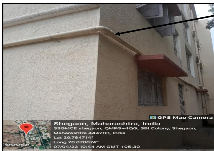
Rain Water Carrying Pipe:
