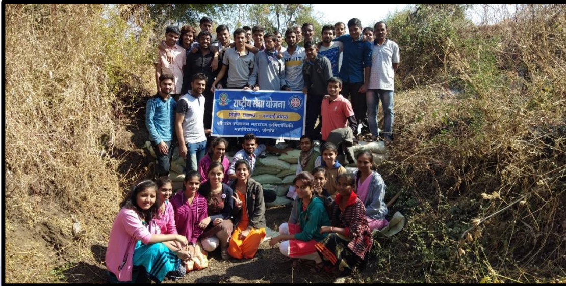
Small scale dam construction work
