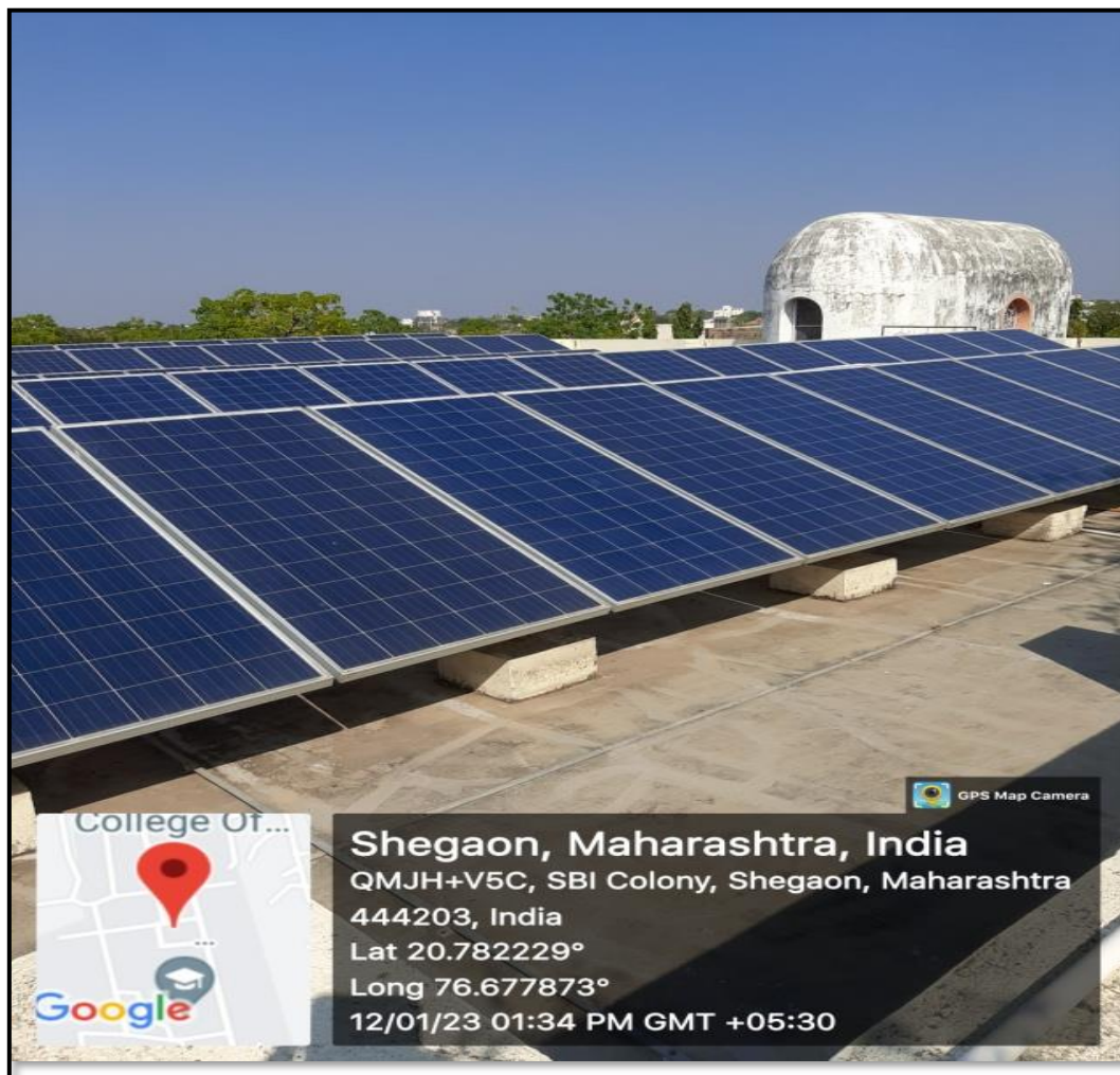
Installation of Plant at the rooftop of Faculty Building
