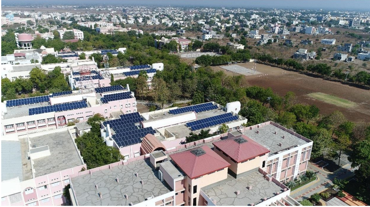
Installation of solar panels across all departments
