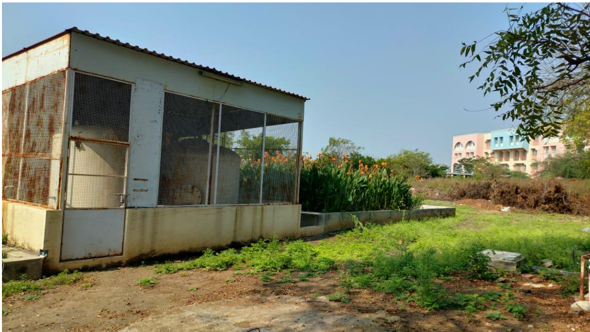
Sewage Treatment Plant
