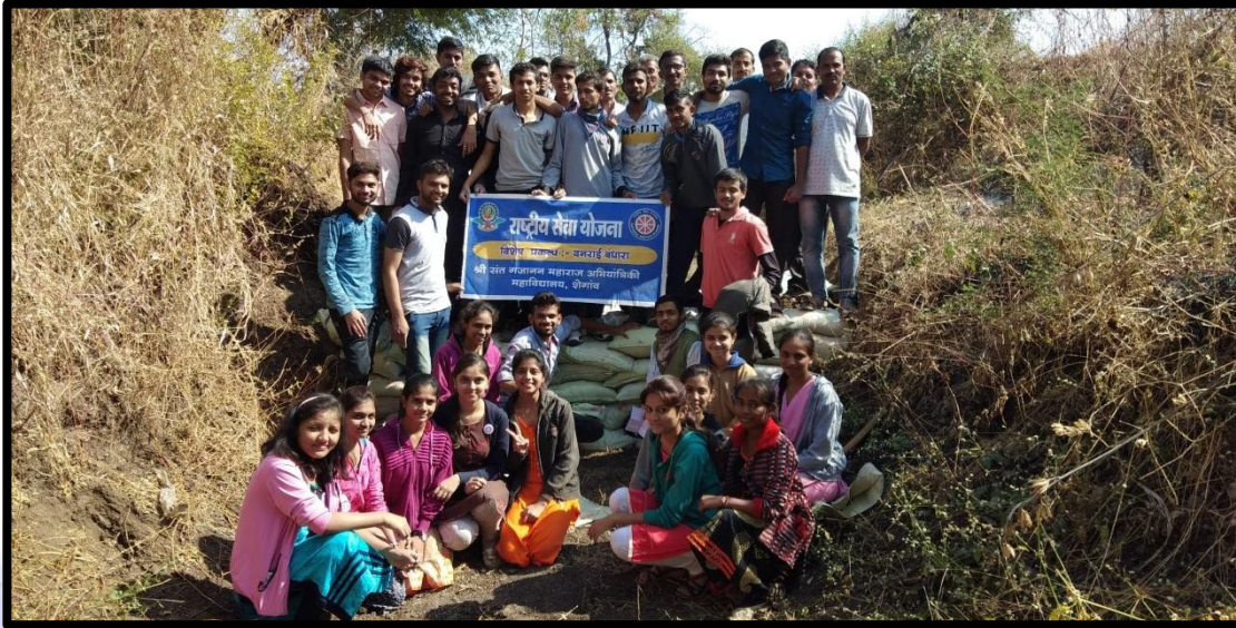
Small scale dam construction work 19th December 2018
