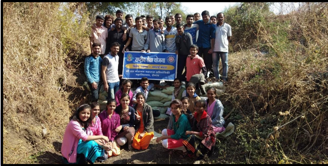
Small scale dam construction work 19th December 2018
