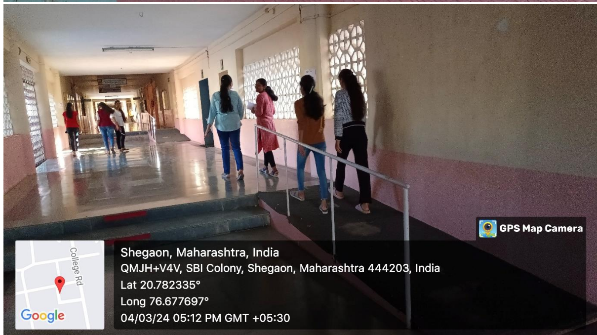
Railing at academic building
