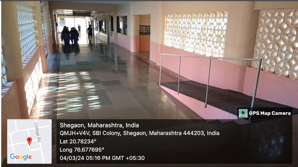
Ramp with Railing at academic building
