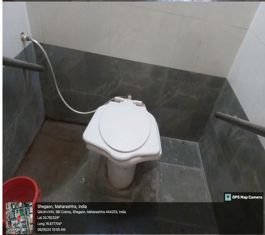
Toilet with railing
